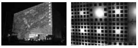
Fig. 14: Green Pix, sustainable curtain wall by Simone Giostra & Partners and Arup, 2008 (left). The coloured LED display with the first photovoltaic system integrated into the glass curtain wall (right).
